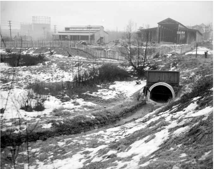
Image 13. Photo title: “China Creek, East 7th Avenue & Glen Drive.” Photo taken 1950. Vancouver Public Library Accession Number: 81146. This photo shows the outfall from the China Creek Trunk Sewer at East 7th and Glen Drive. Note the woman and child at the mouth of the sewer.
