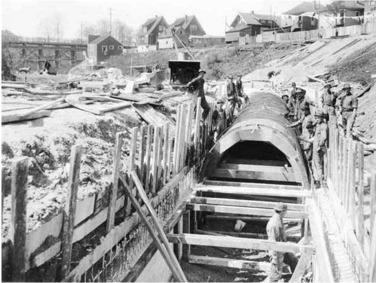
Image 11. Photo title: “Sewer construction at China Creek.” Photo taken 1913. City of Vancouver Archives Str P270.05. This part of the sewer is below the Broadway trestle, showing the depth of the ravine in which China Creek ran.
