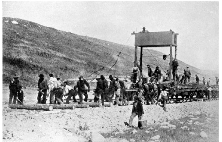
Track laying machine. Courtesy of the Canadian Pacific Archives
