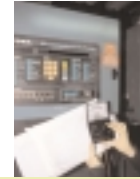
above: calibration of equipment during commissioning
