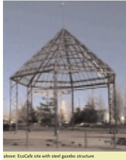
above: EcoCafe site with steel gazebo structure
