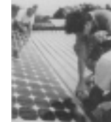
above: workers building a photovoltaic array
