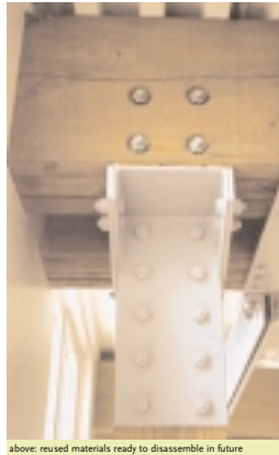
above: reused materials ready to disassemble in future
